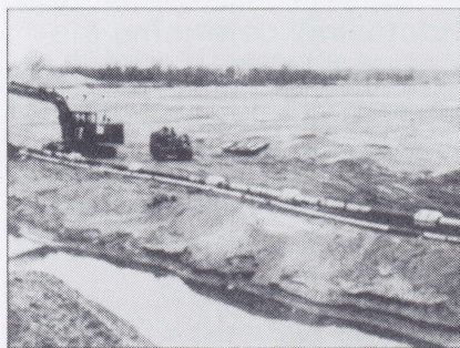
Fig. 2. Bolt-on concrete weights, which weighed 830 lb each, were not sufficient to prevent the pipeline from coming out.
