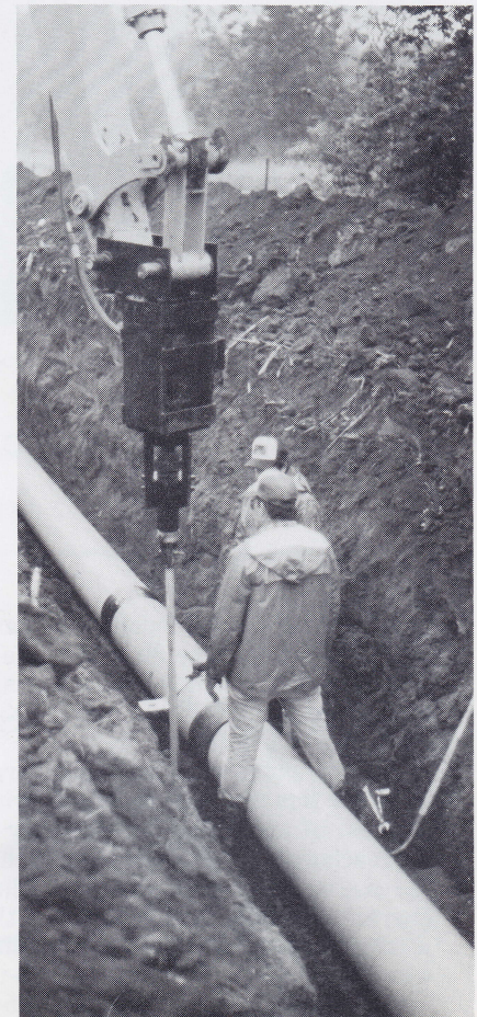
Patented anchor installation tool mounted on backhoe. Device can also be mounted from tractor sideboom. Unit connects hydraulic system of either tractor or backhoe.
