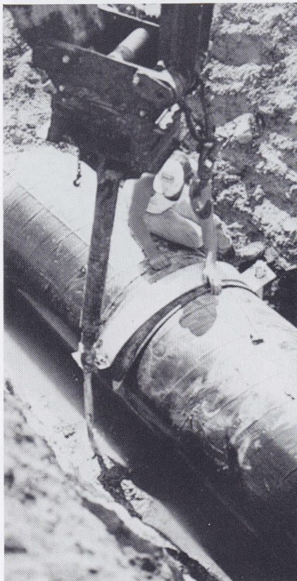
Two anchors make up a set. Once both anchors are installed and tested, a pipe strap is attached to the anchors. Strap rests on a pad to prevent damage to coating.
