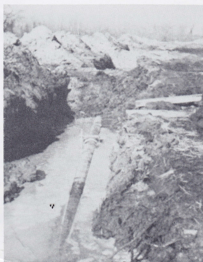
Here is the hook anchor installed on Canadian River crossing job.
