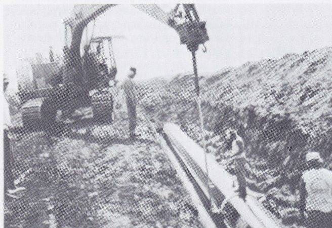
Cat 235 Backhoe used to install anchors on 42" Northern Border Pipeline in Iowa.
